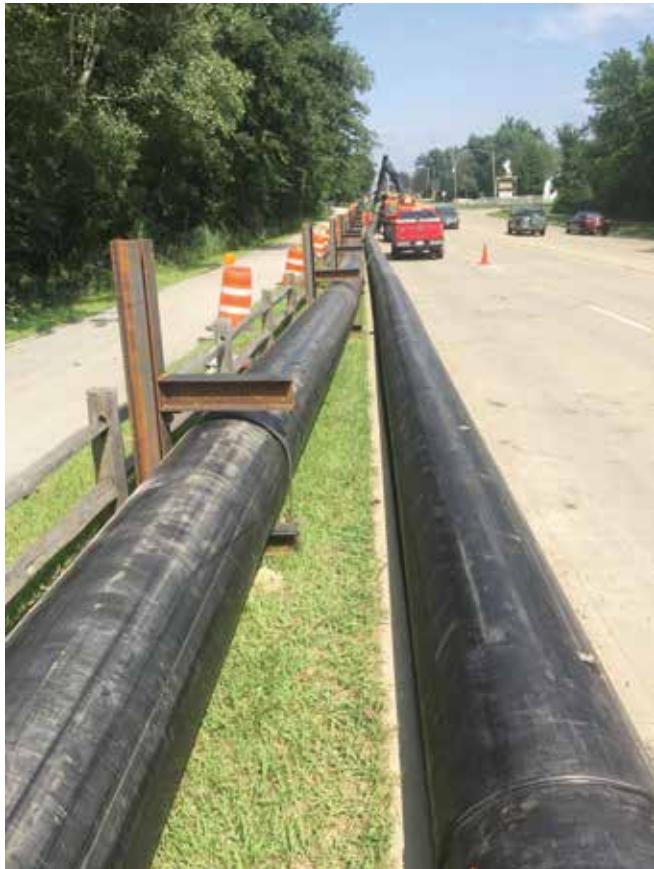
Figure 4. Cantilevered "H" beam used to stack 24" HDPE for bypass
